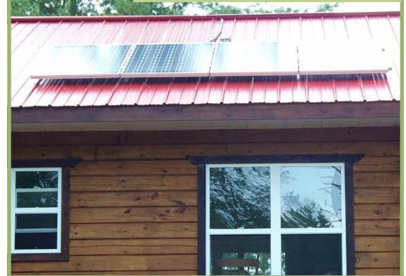
Residential application of a complete Solar Energy System - Solar PV Roof Top Panels
